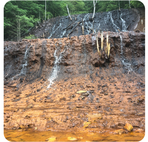
This untreated mine drainage blowout flows into the Casselman from the Shaw Mine complex on the hill above.
