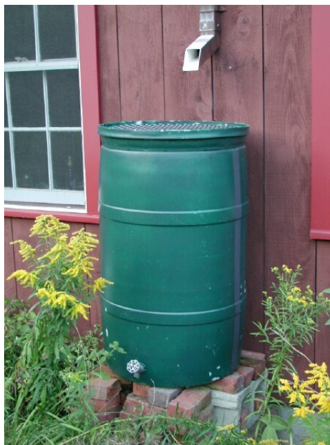
Above: A rainwater collection barrel. Photo courtesy of the city of Winston-Salem, NC.
