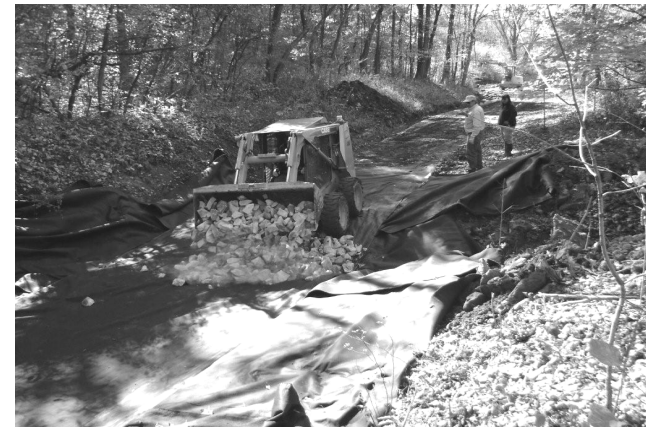
MWA's Trail Committee overseeing construction on the Donegal extension.
