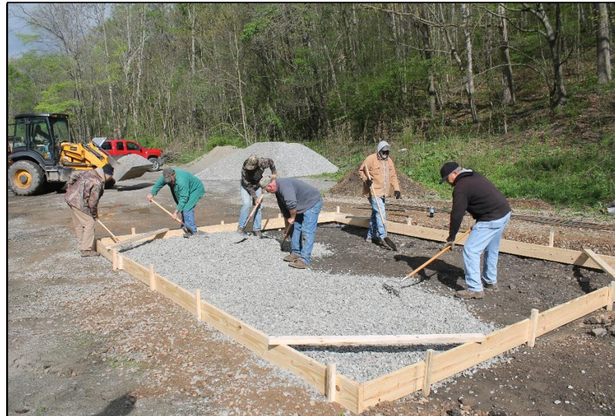
Volunteers installing a handicapped parking space at one of the trailheads for the Indian Creek Valley Trail.
