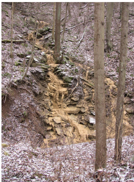
An unnamed tributary to the Yough showing erosion and sedimentation from the Curry site. For color photos visit our website.
